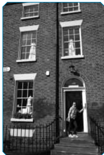
A typical Georgian House.
